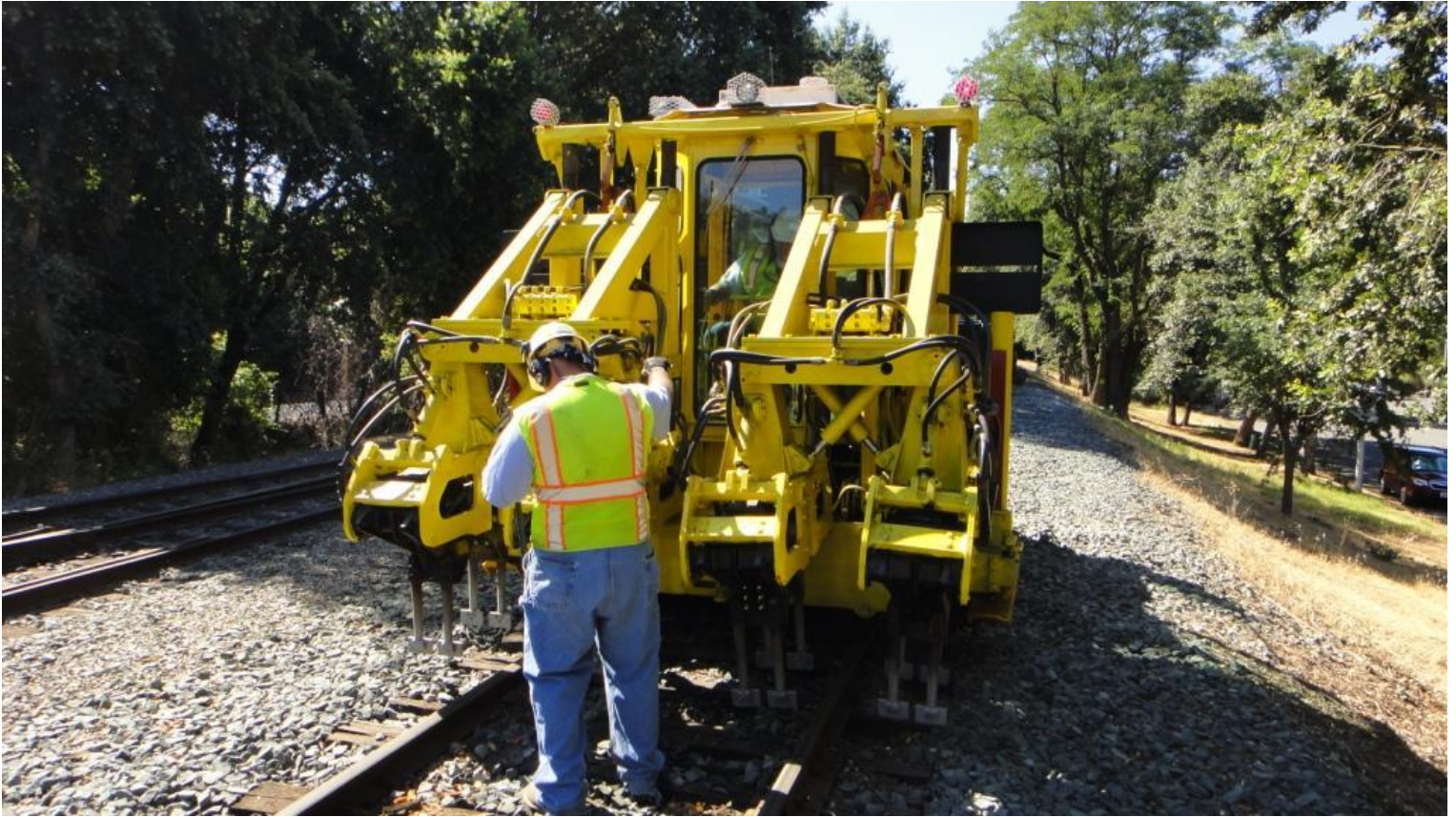
Mike F. guides Harry in the tamper as the tamper tamps the track at its new level
