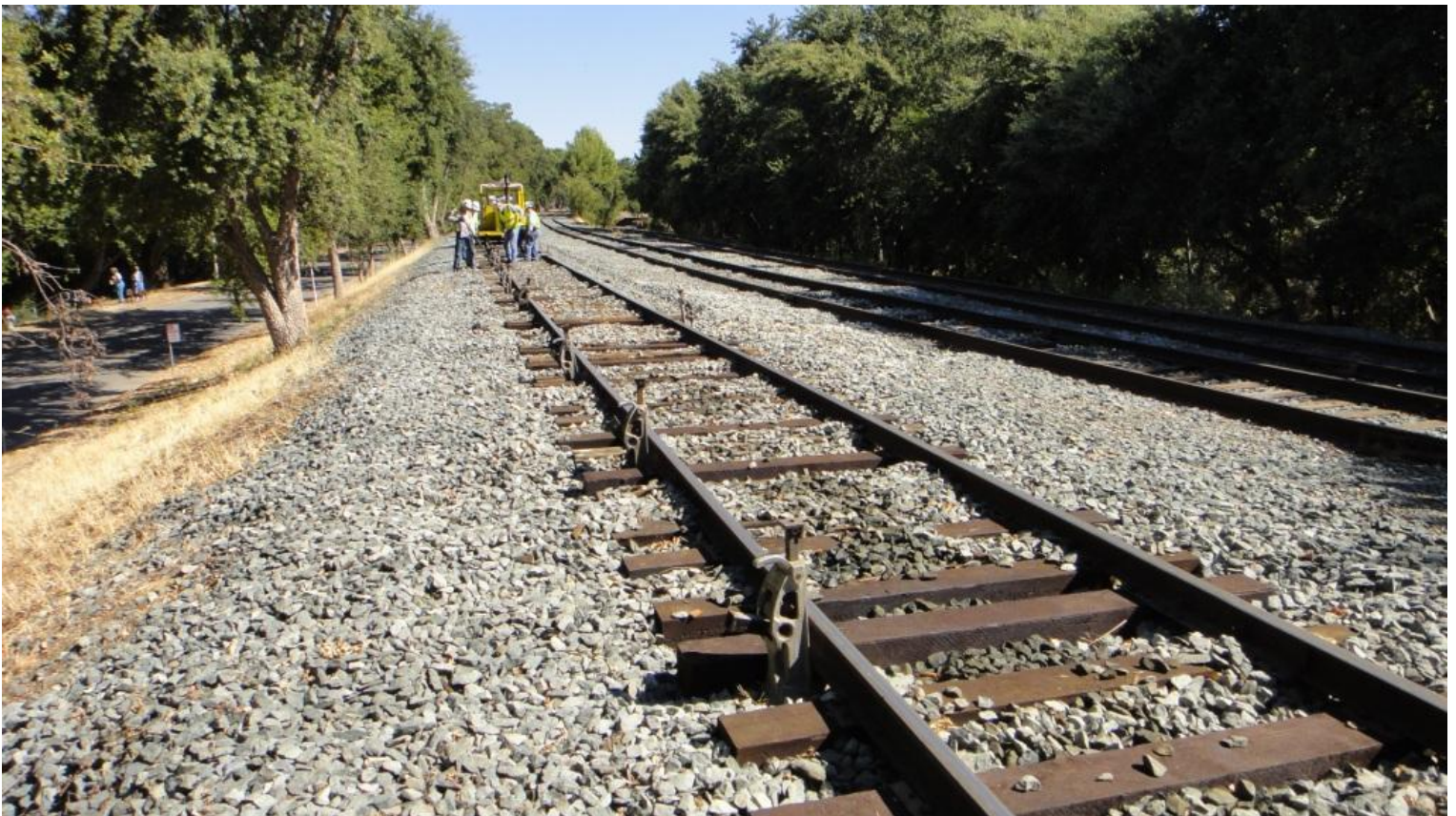
Track-jacks standing at attention like soldiers
