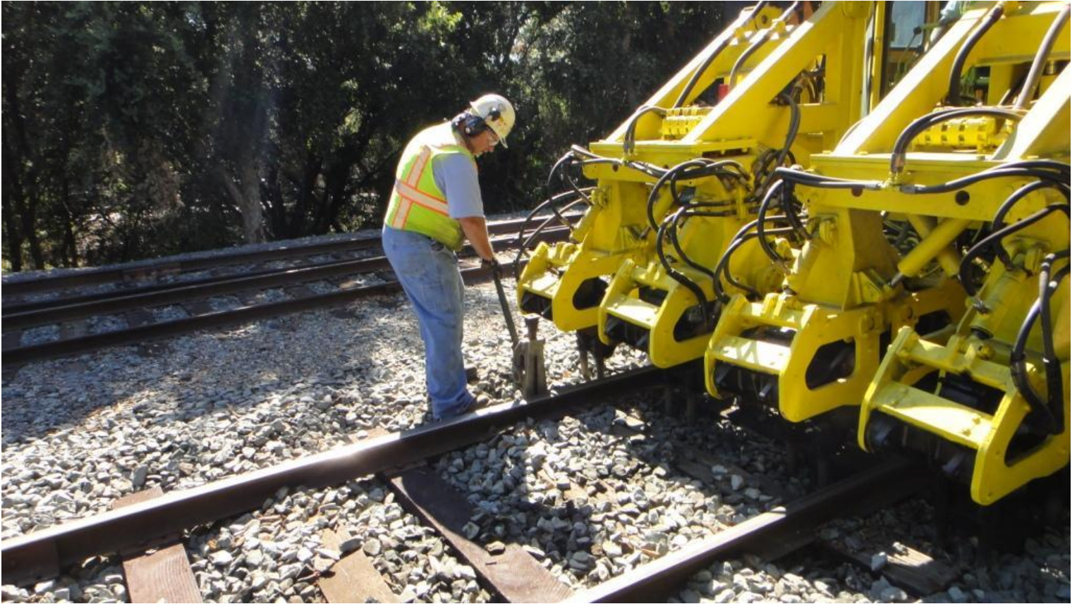
Mike F. removes a jack as the tamper comes in to build support under the track at its new level
