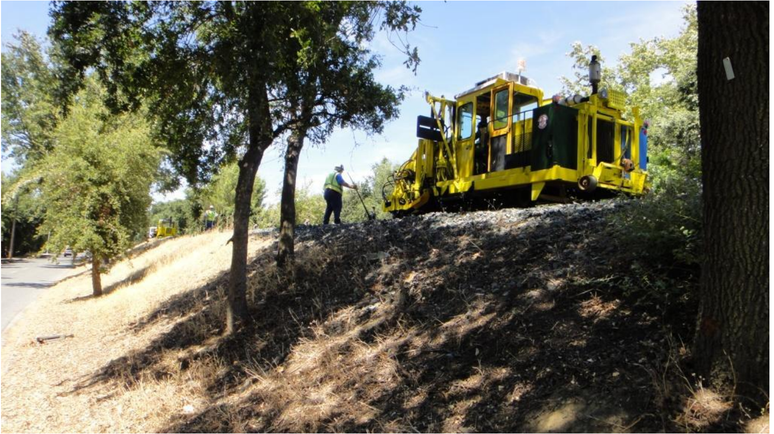
Frank prepares to remove a jack as the tamper approaches
