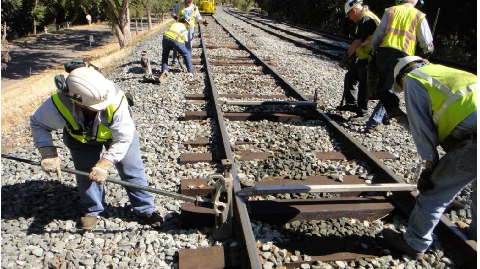
Mike M. checks the level as Heather jacks-up the west rail
