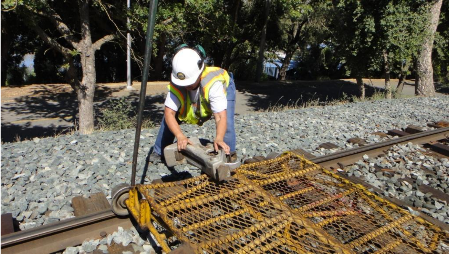
Pam removes a jack from the Nolan Track Cart at the next section of track to be leveled
