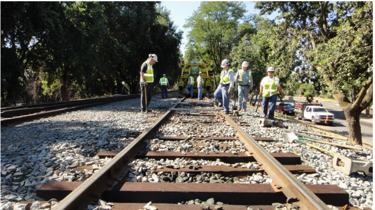
Using track-levels, the team deploys track-jacks along the low west rail
