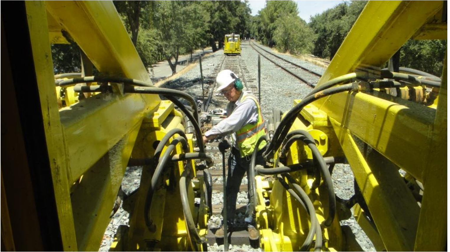
Steve guides the tamper from the ground to make sure that no ties are accidentally "speared"...
